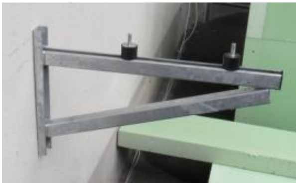
Figure 12: Wall bracket side view
